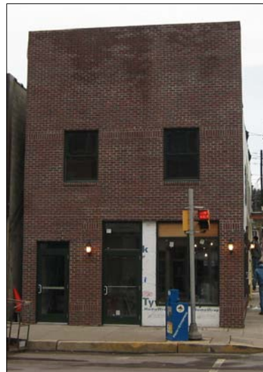
NEW MAIN STREET ELEVATION UNDER CONSTRUCTION
